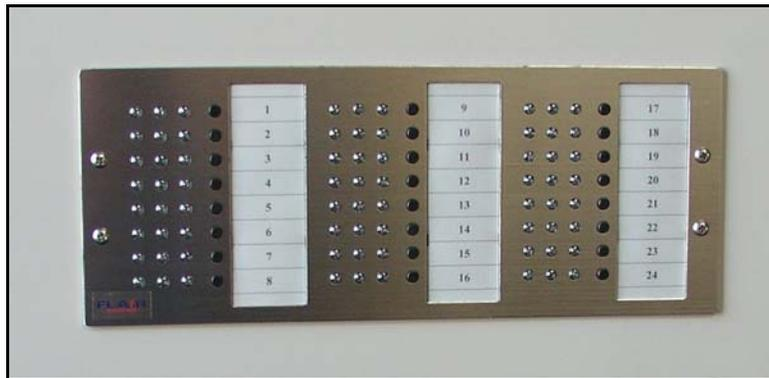
The 561A Multi-Zone Annunciator is ready to use from the factory. It comes pre-configured with basic factory (default) settings and will work with NC or NO devices with 1K Ohm EOL Resistors.
